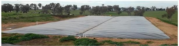
Treated effluent and pond sludge is then pumped to three Sedimentation and Evaporation Ponds (SEPS) which are dried out and desludged annually. The overflow from the SEPS is pumped to holding ponds from where treated effluent is recycled for flushing and irrigated to paddocks.
